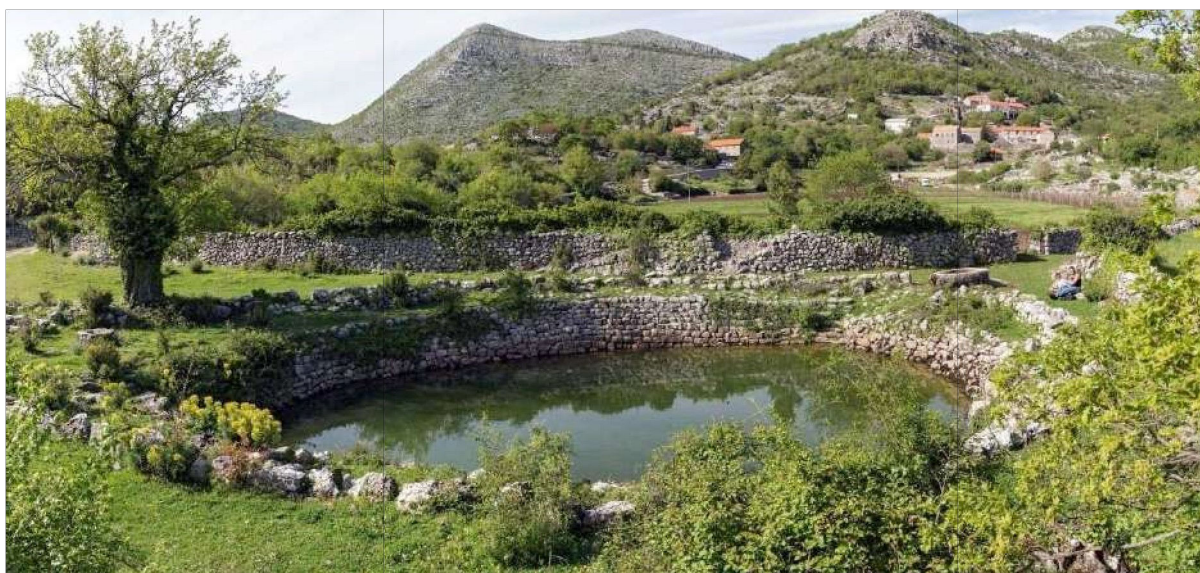
Dry stone pool dans in one of the Konavle village, 17m of diameter
