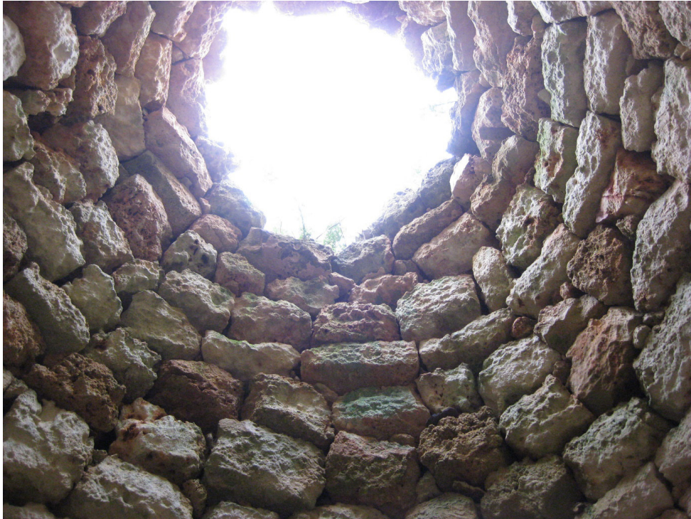
Corbelled vault with part missing.
