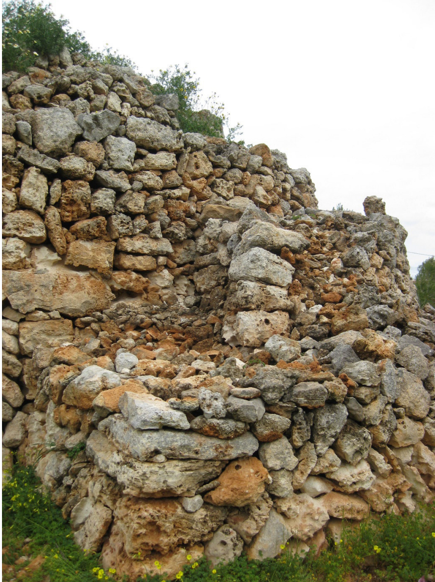
Right side of the entrance with the wall angles to restore.
