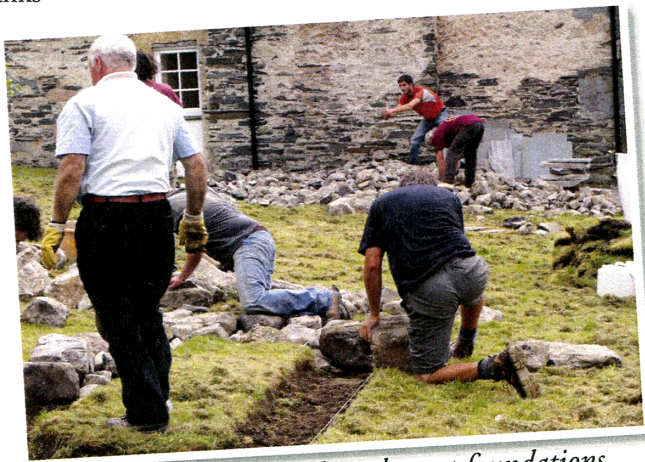
Work starts on building the seat foundations. Photo by Alison Shaw
