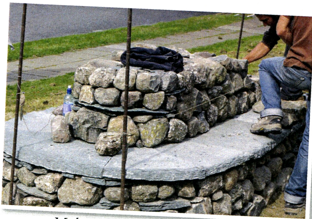
Making sure the lines are straight. Photo by Alison Shaw
